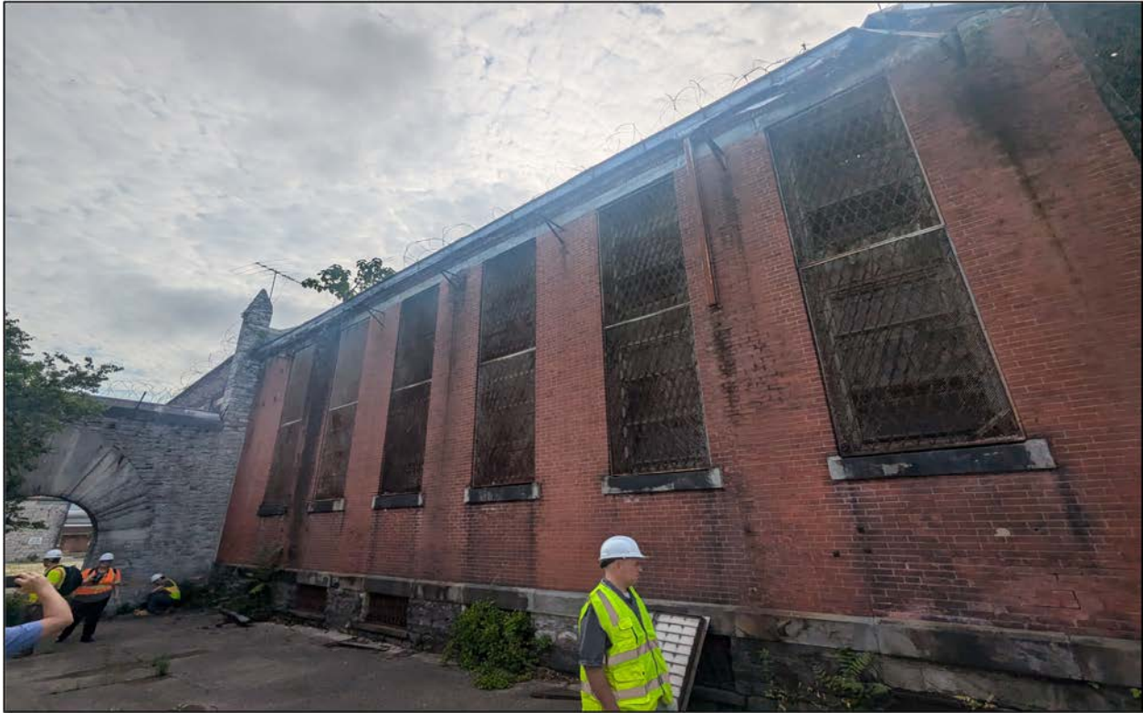
Figure 17. Phase III exterior from west courtyard
