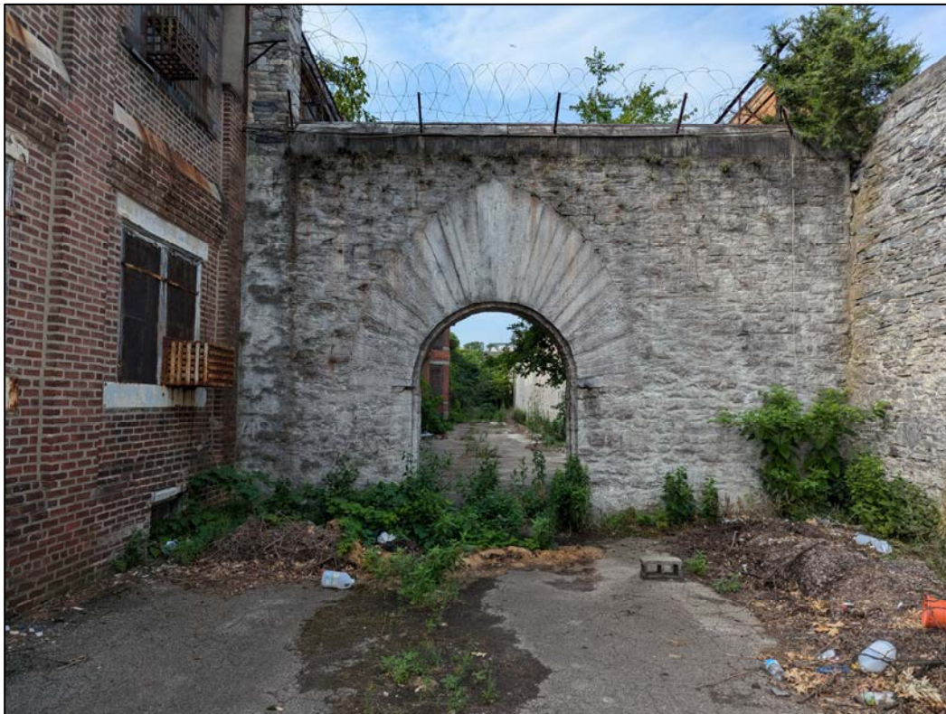
Figure 9. East Prison Wall Arch, View South
