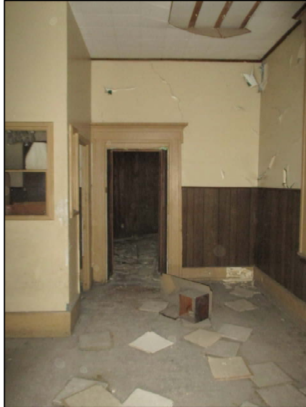
Figure 11. Phase I Interior
