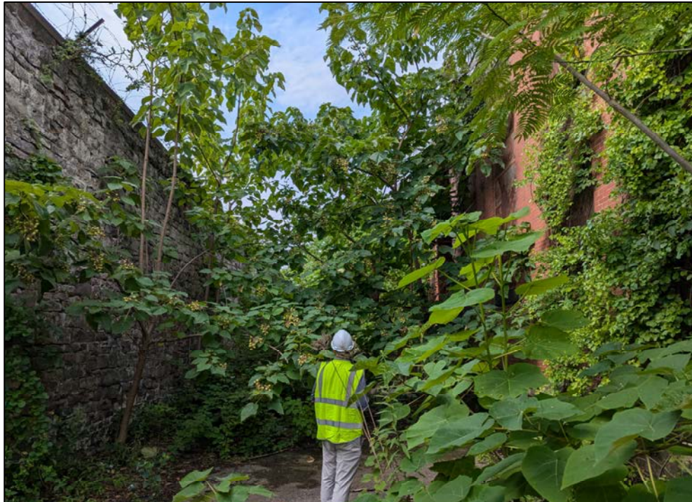
Figure 7. Vegetation within the east yard
