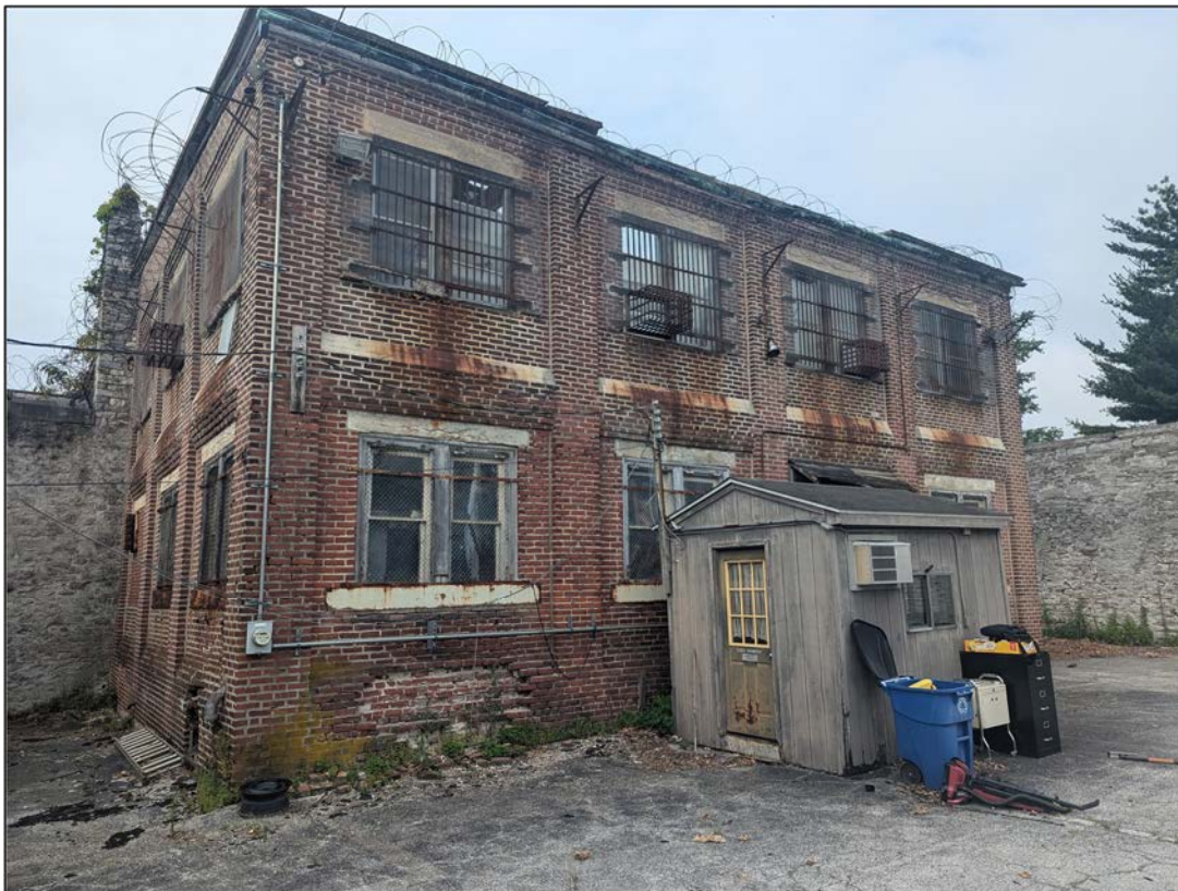
Figure 20. Phase IV exterior
