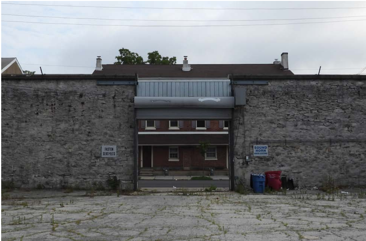
Figure 21. Marshall Street roll-up gate
