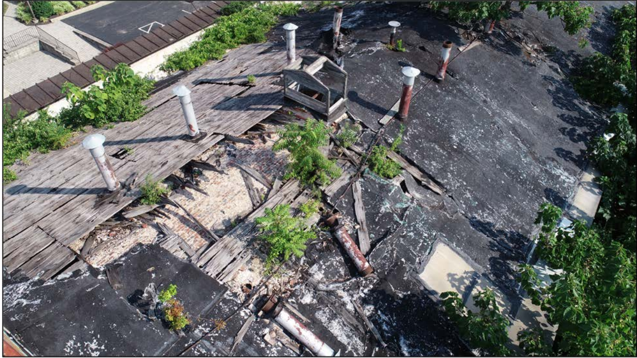
Figure 14. Phase II Roof
